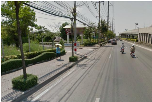
Figure 2. Sidewalk of School A
